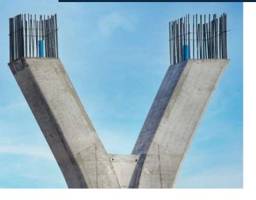
Steel reinforcement provides the necessary tensile strength to support these loads, allowing for taller and more dramatic designs. In addition, the flexibility of steel reinforcement means that it can be shaped and manipulated into a wide variety of forms, making it ideal for complex architectural designs.
