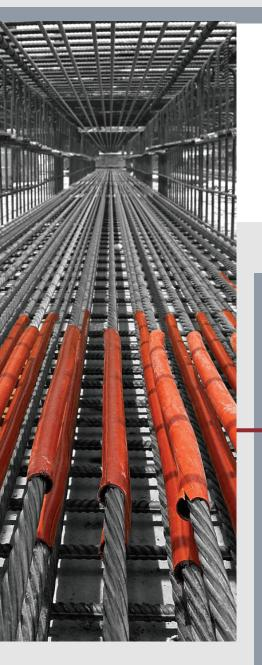
Prestressing strands are high-strength steel wires that are placed in the concrete before it is poured.
